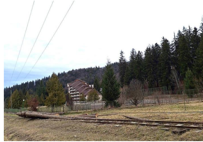
The hotel structure that appeared after deforestation
